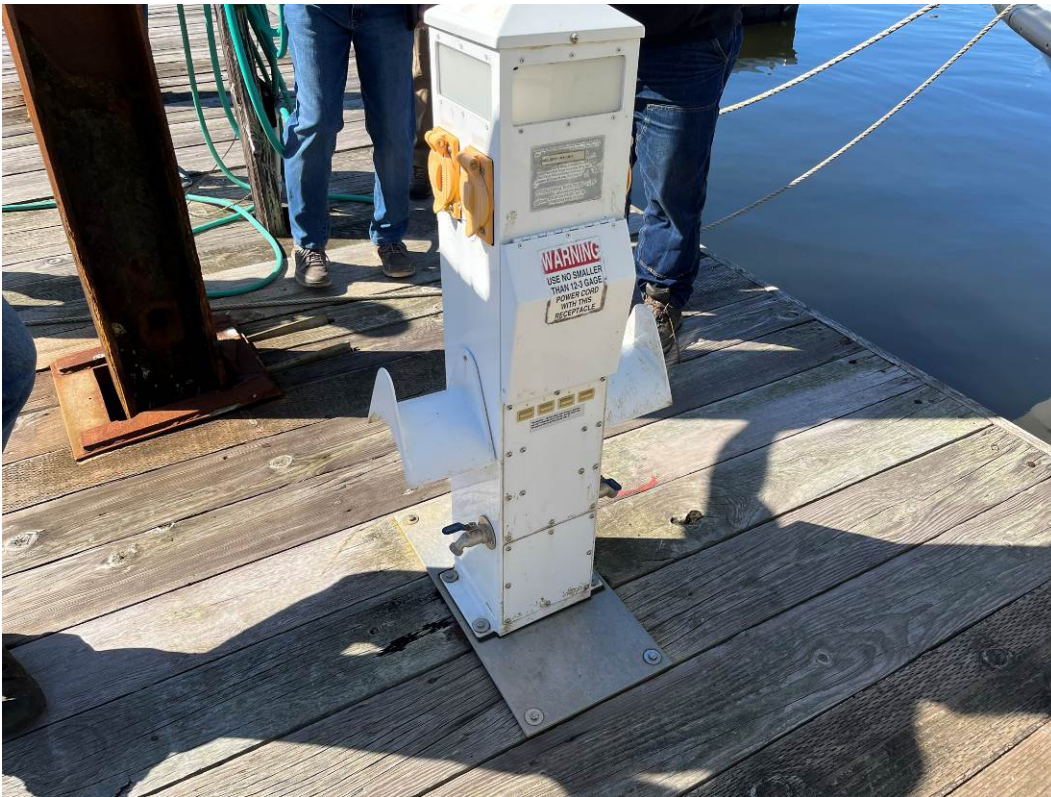
Photo 15 – Utility Pedestals with Potable Water
