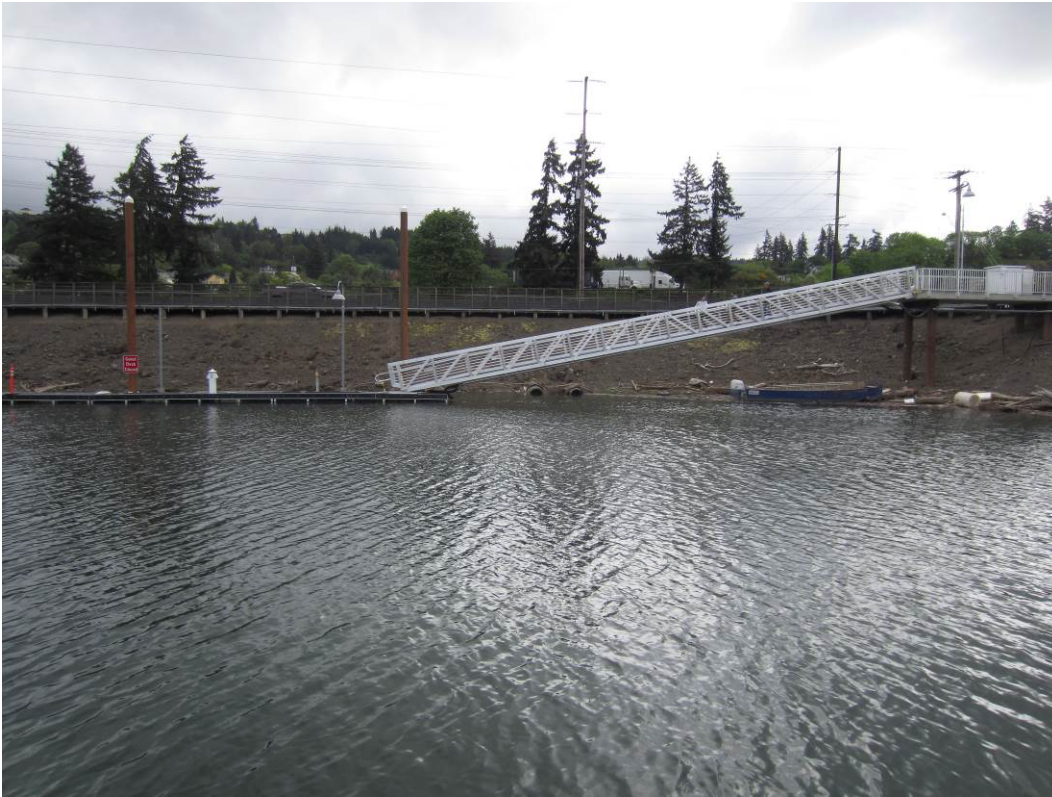
Photo 17 – 80-foot Long ADA Gangway Ramp (Port of Kalama)
