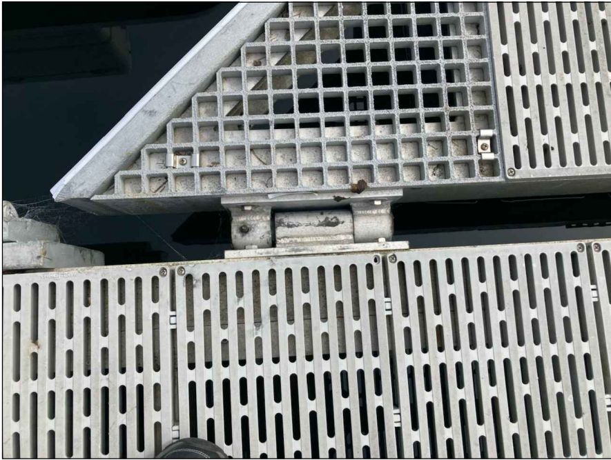
EXISTING HINGE CONNECTION PHOTO
