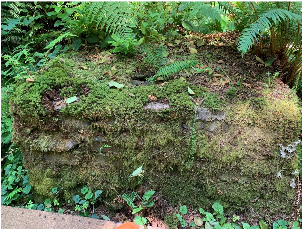
Figure 8. Close-up view of courses of tabular basalt in south wall of still.
