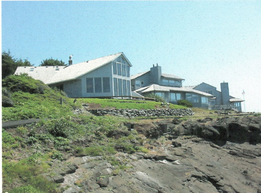
Photo 1 - Looking south-southwest toward site. Note the rockery wall.
