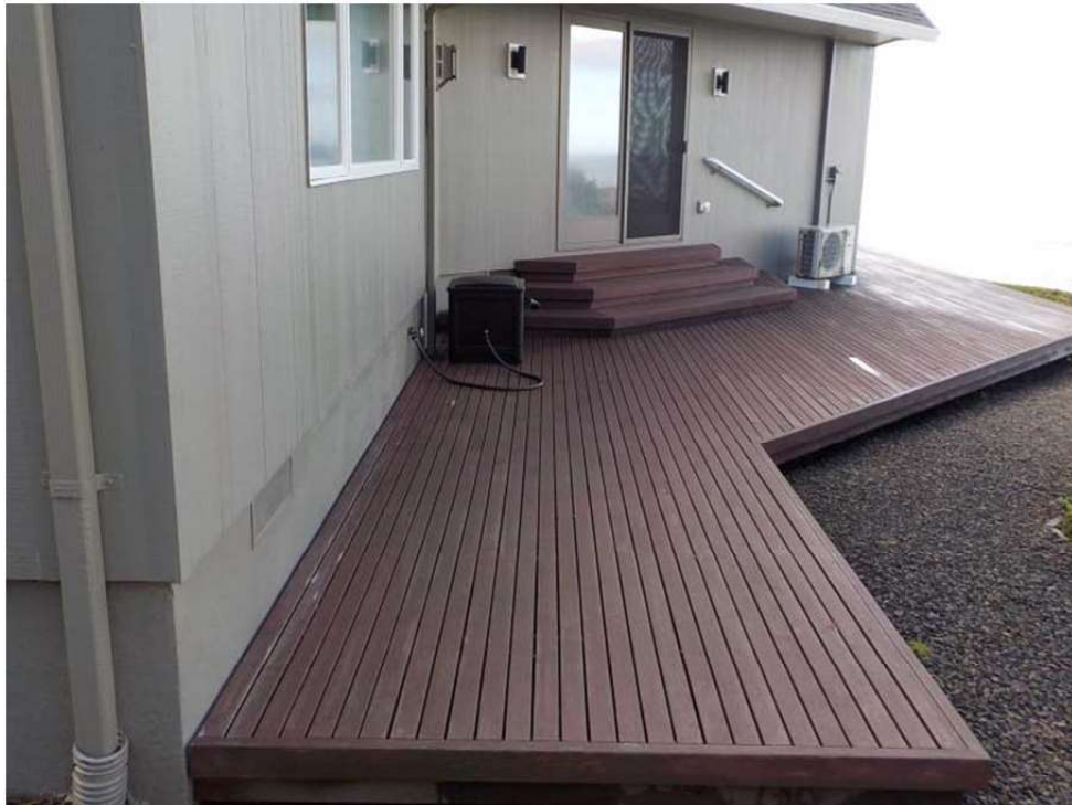
Photo 4 – View of the northern portion of the existing deck.
