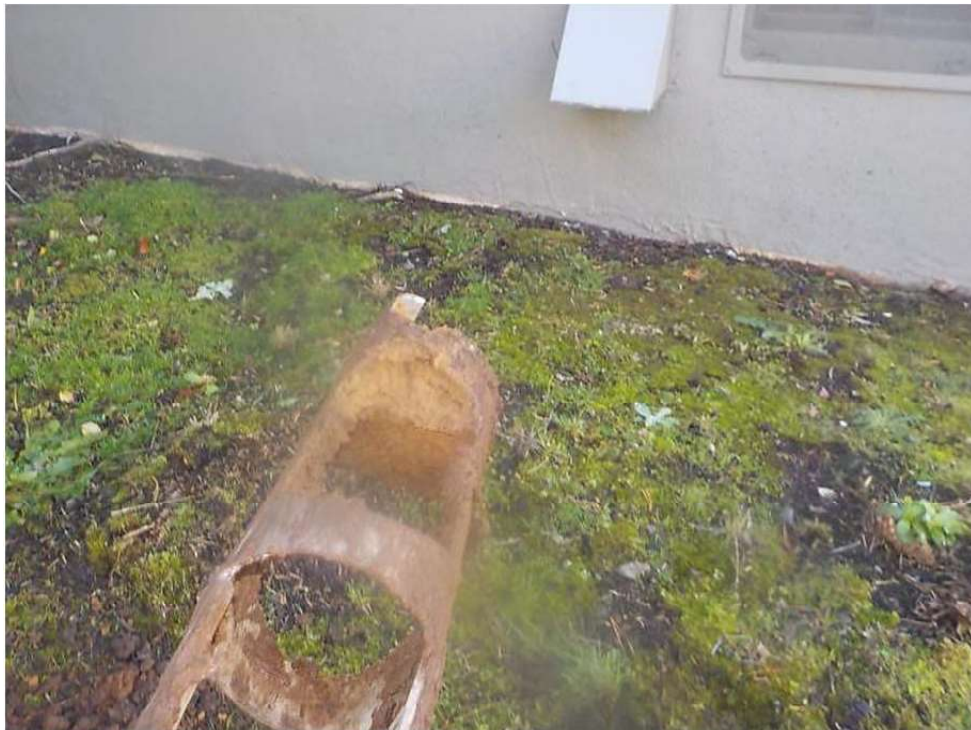
Photo 6 – Close-up view of the stiff clay soil encountered in Boring B-1.
