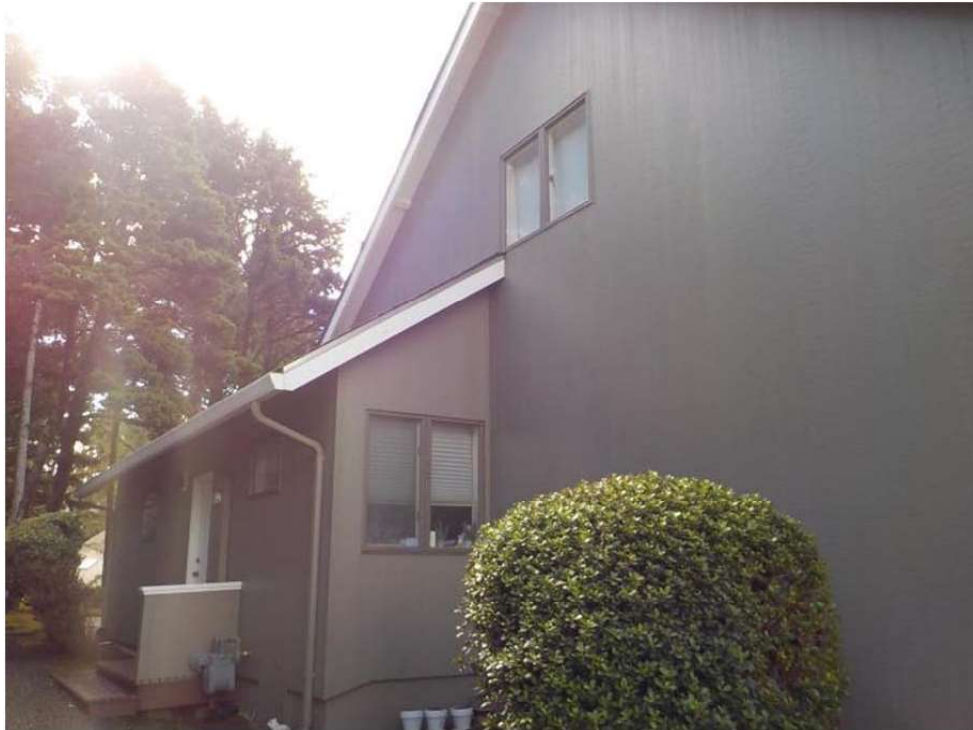
Photo 2 – Southerly view of the area of proposed construction.
